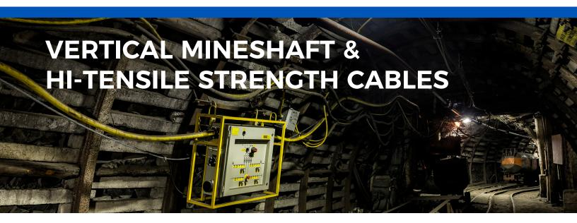
Shawflex Vertical Mineshaft cables are designed to prevent cable core slippage and are suitable for use in vertical installation and for environments that require self-supporting lengths. Typically used in Mineshafts, Tall Commercial Buildings, Inclined Tunnels and Vertical Cable Trays.
